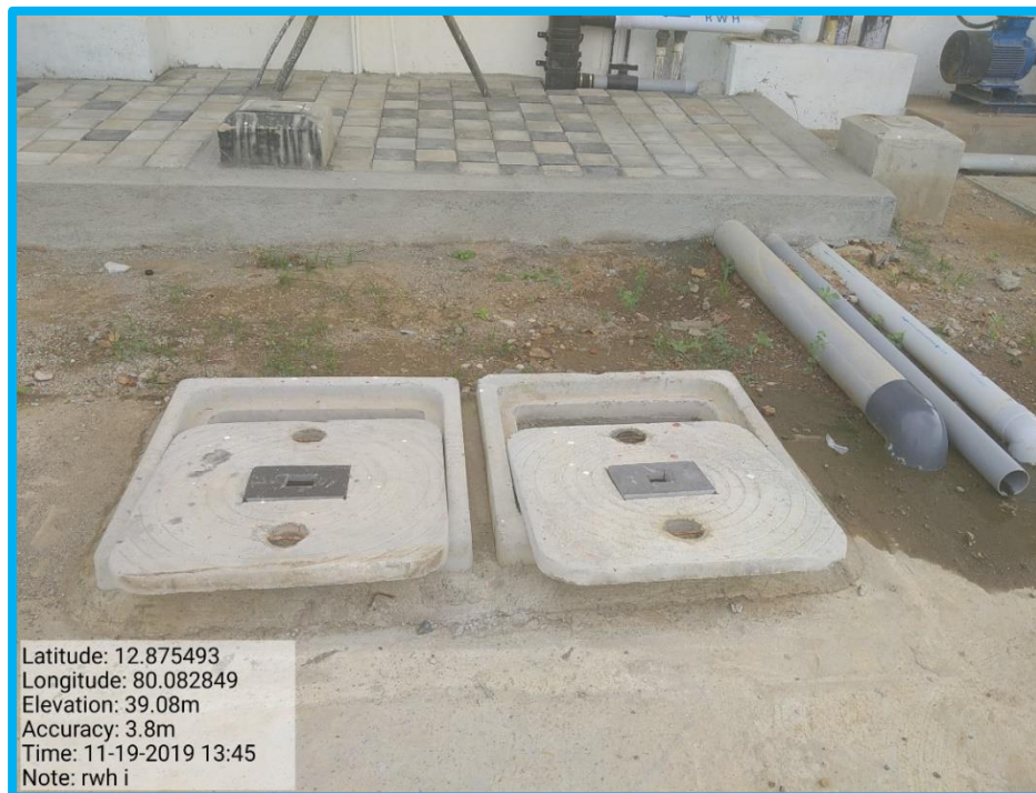
Figure VI (5.4) – 14: Rainwater collection sump (architectural block)
