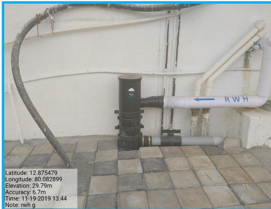
Figure VI (5.4) – 13: Filter unit in rainwater harvesting system (architectural block)
