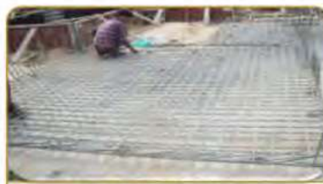
Figure 2 : View of CPAC Coated Reinforcement Rods at Site
