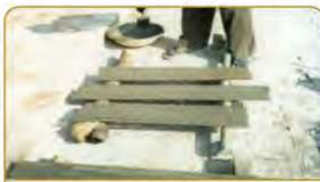
Figure 1 : Application of Cement Polymer Anticorrosive Coating (CPAC)
