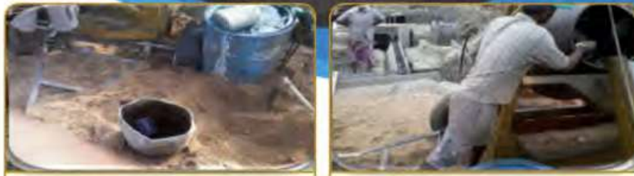
Figure 3 : Preparation of Corrosion Inhibitor Admixed Concrete
