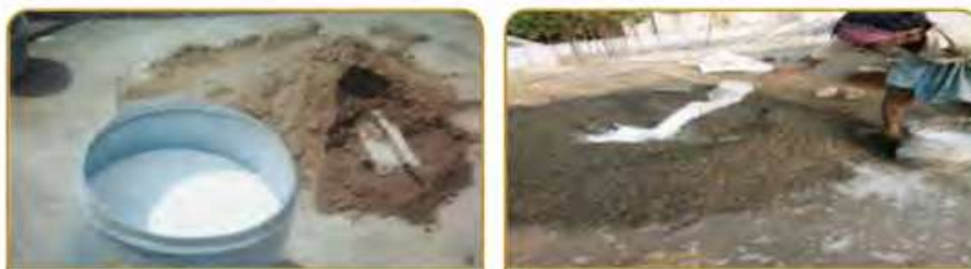
Figure 4: Preparation of Polymer Modified Concrete
