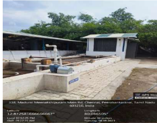
STP 100 KLD capacity Increased in Men's Hostel
