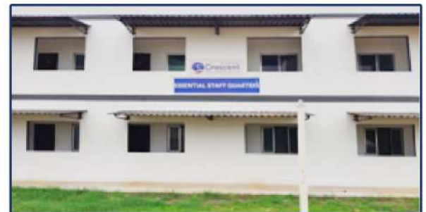
Building Units planned and executed using Glass Fibre Reinforced Gypsum (GFRG) Panels by Faculty and Students of Civil Engineering Department
