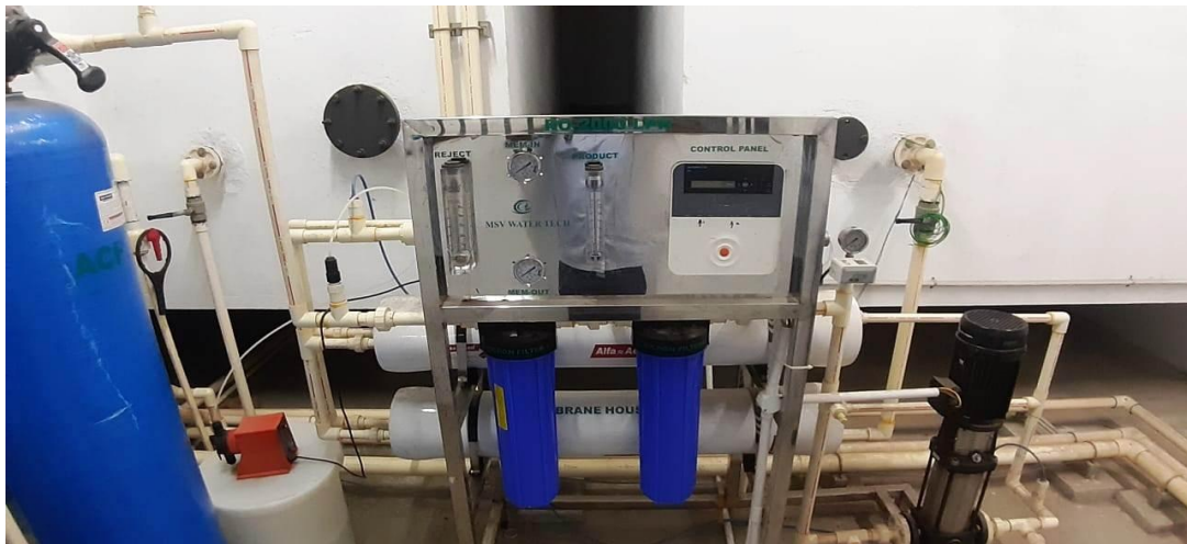
ARCHITECTURE BLOCK RO PLANT
