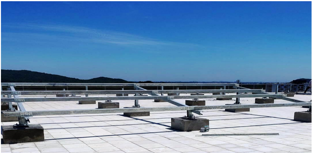
100 KWP ROOFTOP SOLAR PLANT UNDER CONSTRUCTION
