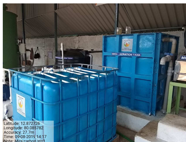
Mira carbon sewage treatment plant
